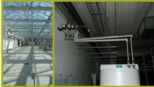
Start Frame work and pipe runs
