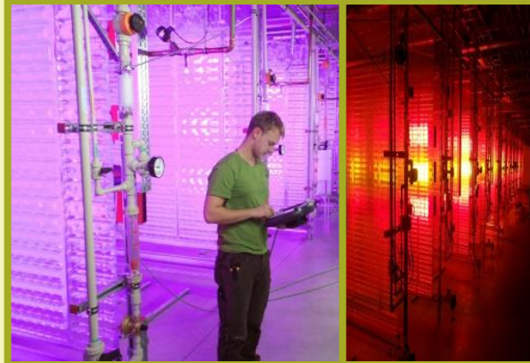
Start-up and Testing Completed
